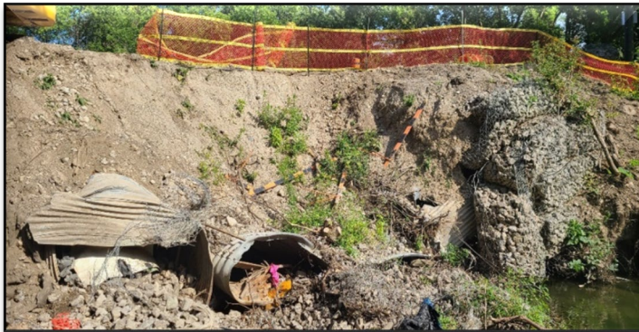
Pedestrian Bridge Bank – Emergency Repair
